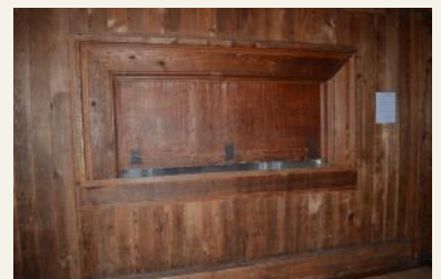
Below: Serving window from prep area to main hall.
